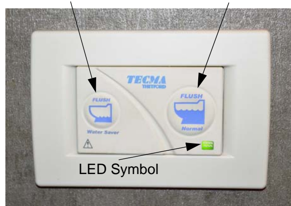
Wall Switch/Controller (Located on wall near toilet)
