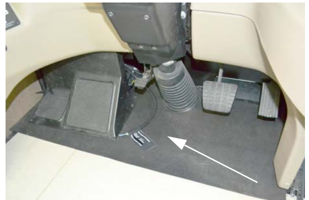
CB Power Wires -Typical View
